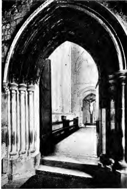
48. South Doorway, St Etheldreda.
